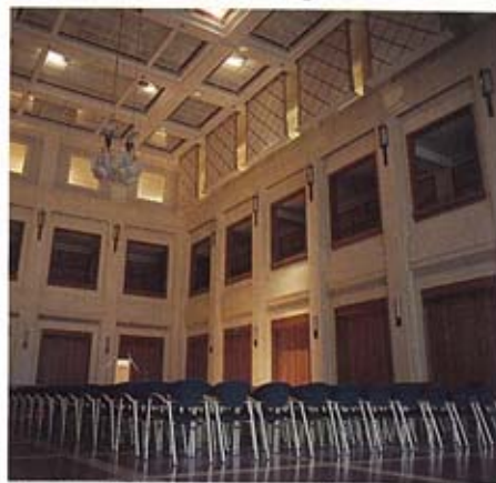
The Cabot Hall showing acoustic banners and loud-speaker cluster.
