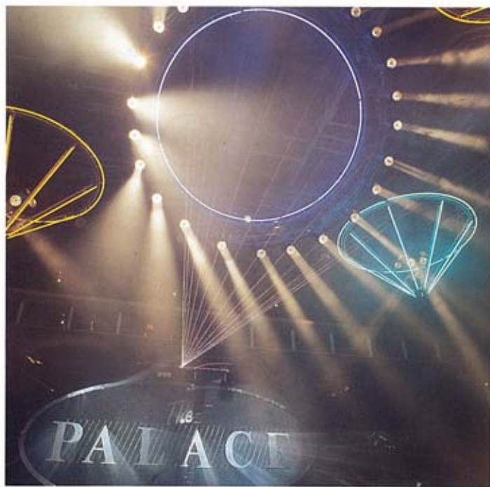
Two neon circles with pinspots around the perimeter arc down to provide movement.
