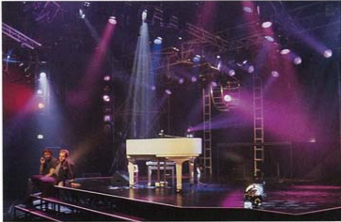
Amongst the lighting on Stage C, Rod Litherland has added Cosmo balls to throw moving streaks of light across the cyc.
